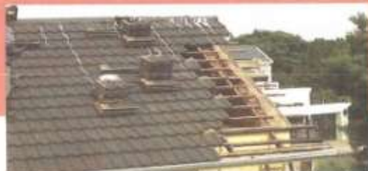
Where necessary, roof is opened and purlen battens replaced
